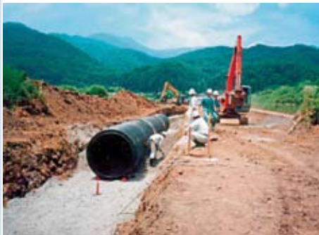
Large-diameter plastic pipes for waste water disposal are on the increase worldwide.
