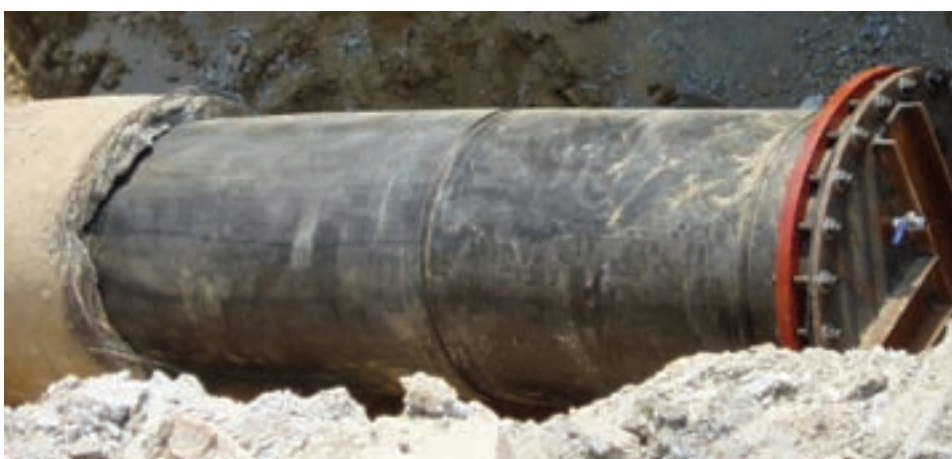
New PE lining pipe in position
