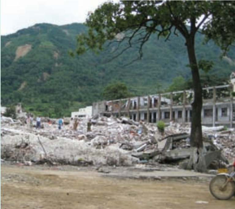
Beichuan High School, reduced to ruins, as a result of the Sichuan earthquake in May 2008
