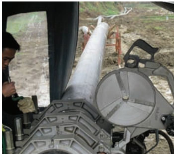
Butt welding the lengths of PE pipe together
