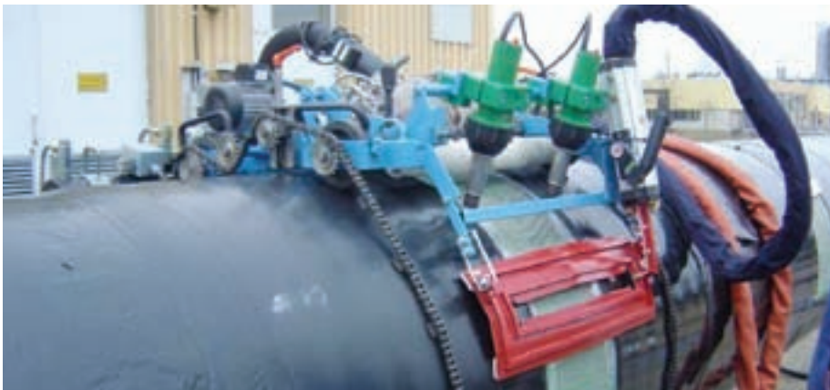
The field jointing machine undergoing testing in Finland
