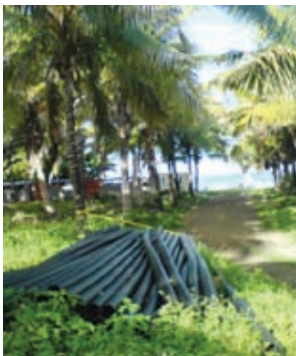
PE pipes ready for installation in the island paradise
