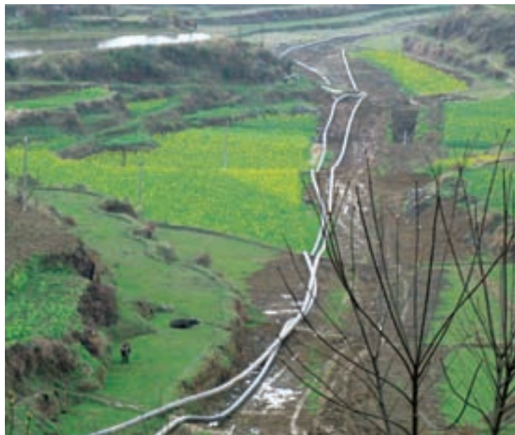
The pipelines lying across the landscape
