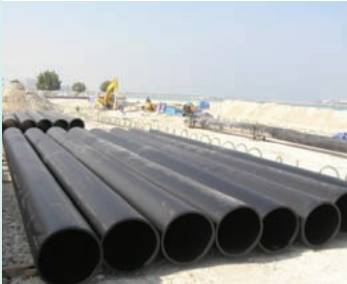
PE pipes ready for installation on Abu Dhabi's new beach
