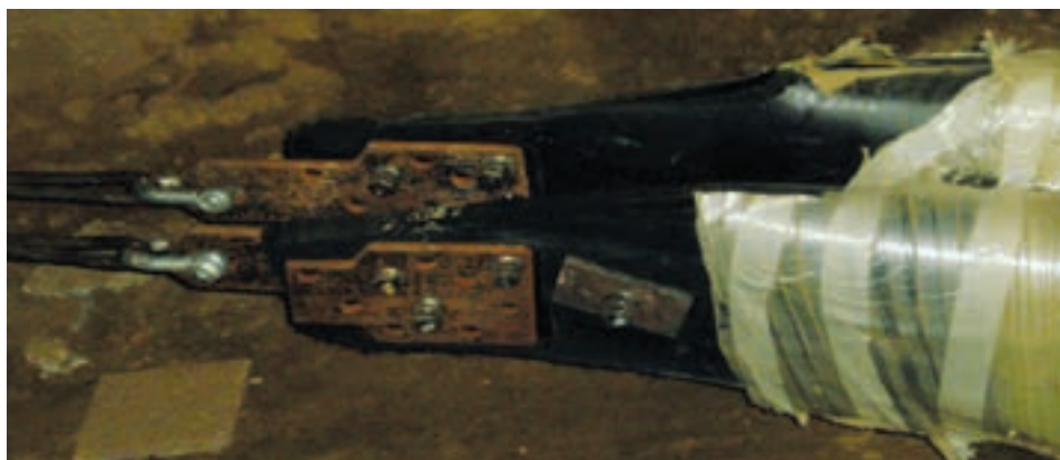
Folded and strapped pipe pulled into main
