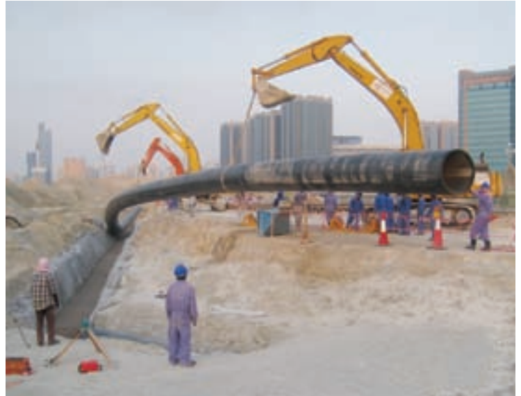
Installing the large diameter PE drainage pipe under the sand
