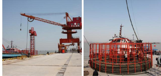
The cable being lowered onto a barge for transportation to the offshore installation site at the harbour dock of the Hengtong (Changshu) High Voltage Sea Cable Industry Park. (Courtesy of Hengtong Group)
