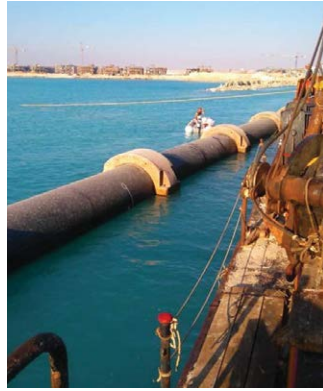
The PE100 pipe string was easily floated offshore.
