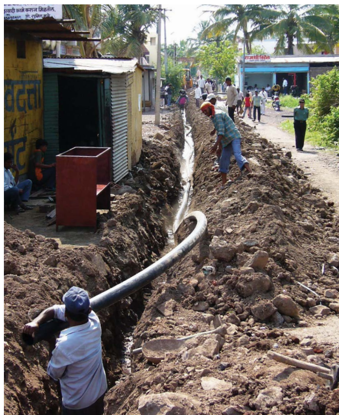
Pipeline installation for the Water for the World project in Malkapur.
