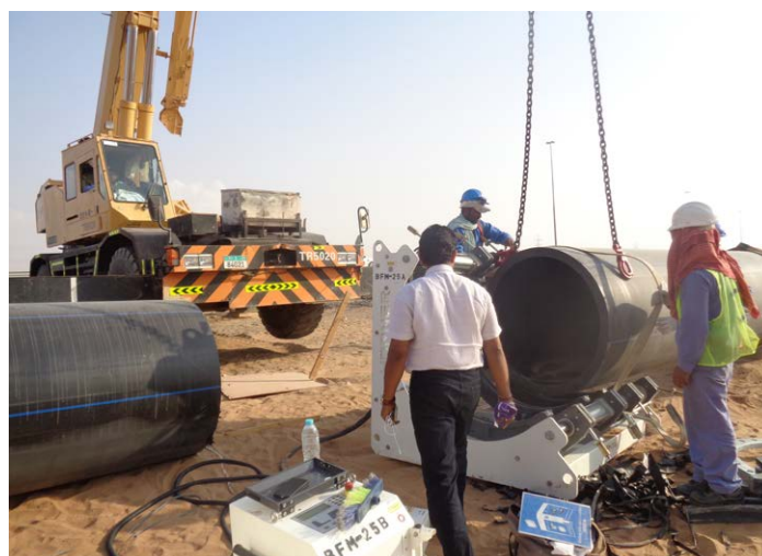
Installation of the pipeline.
