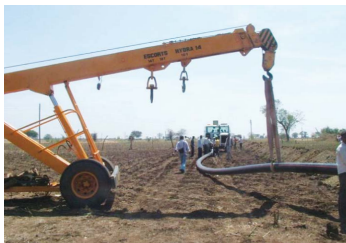
Installation of PE100 pipes by narrow trenching in the Punasa Project.
