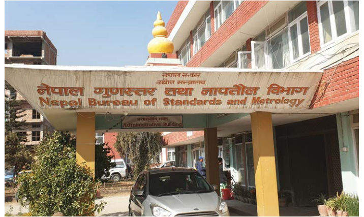
The Nepal Bureau of Standards and Metrology office.
