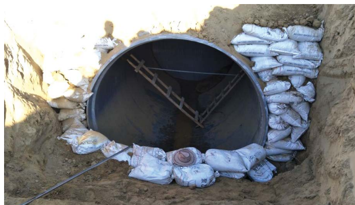
Figure 7. On-site deformation testing of the tunnel. (Courtesy of Minsheng Pipe)
