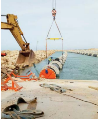
The PE100 pipe string was easily floated offshore.
