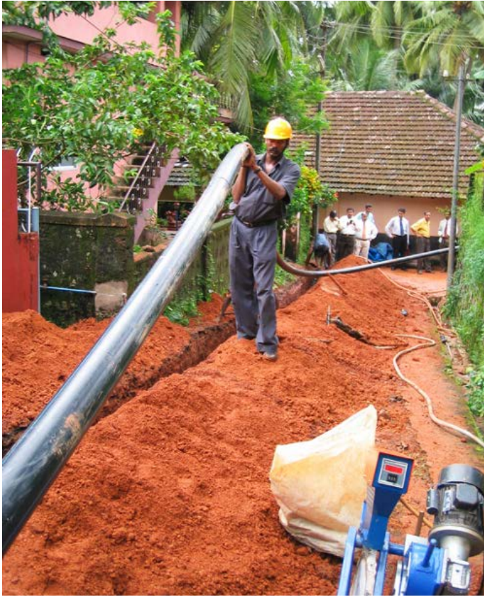
Pipeline installation in progress at Mangalore, Karnataka.
