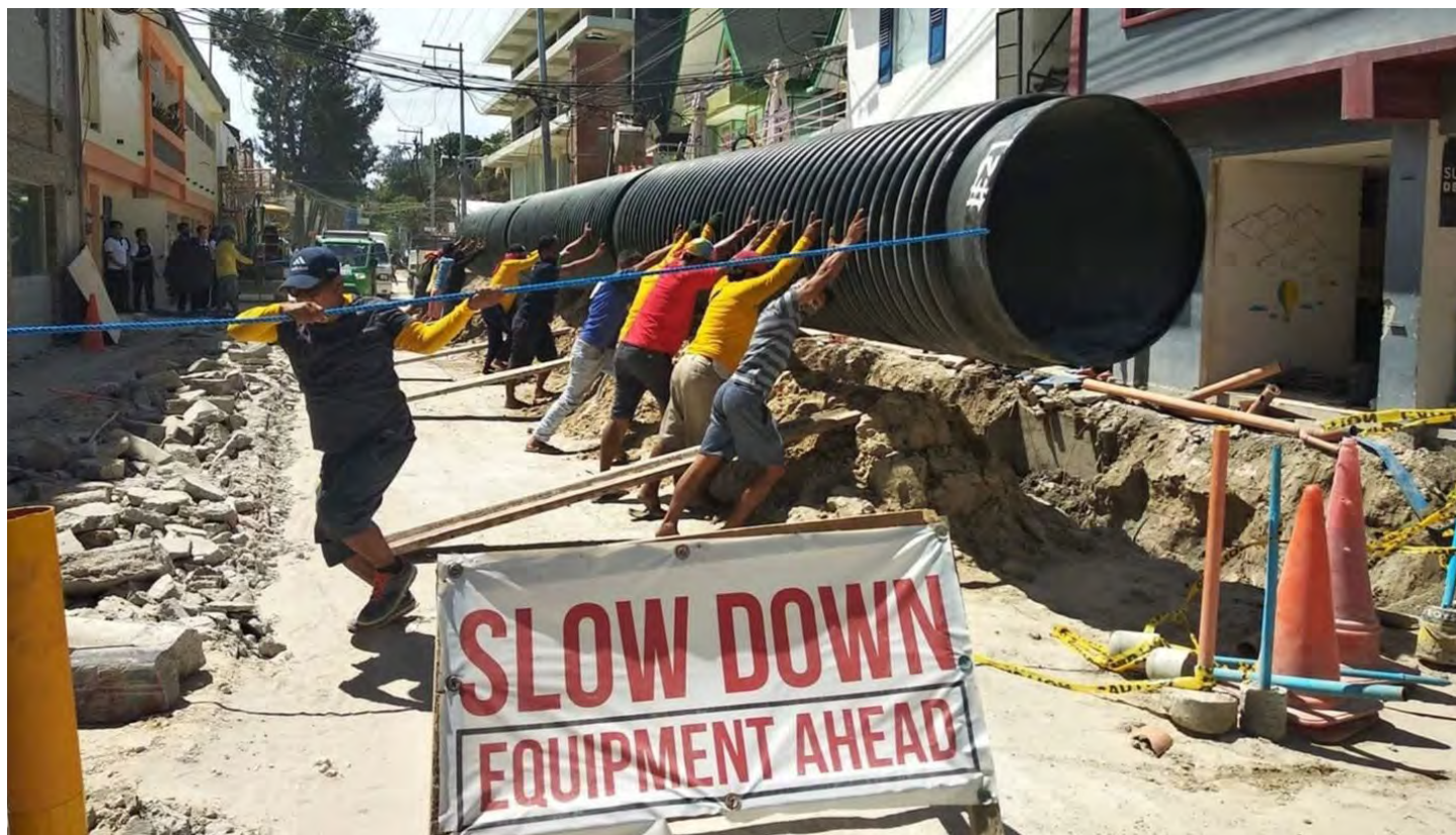
Boracay locals demonstrating the Bayanihan spirit (Communal unity & cooperation to achieve a common goal) during the installation of three pre-jointed DN/ID 1500mm segments.
