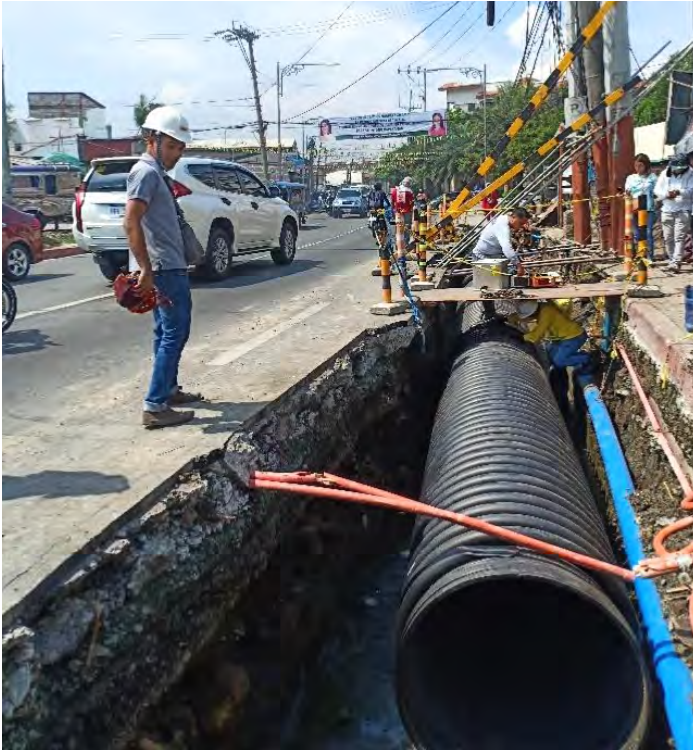
Supervision of pipe laying by Krah engineer.
