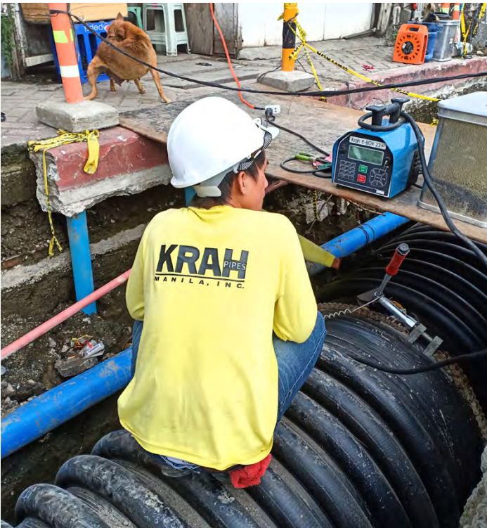
Electrofusion of the pipe sections.
