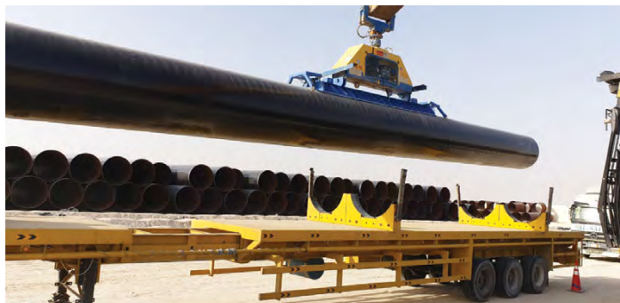
Steel pipes coated with the Borcoat 3LPE system being loaded for the Neom project.
