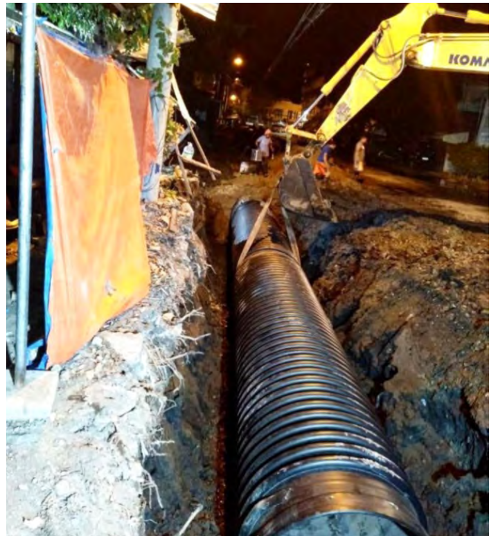
Laying of DN/ID 1000mm along Damaso St. Davao City using light equipment.
