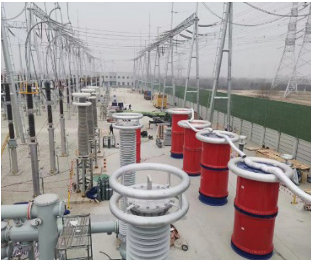
The overhead lines before relocation.
